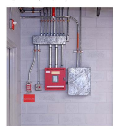
Another common misconception is that Fire Alarm Control Panels (FACP) with built-in fuse/circuit protections do not require external surge protection. The truth is that surge protection built into any individual device will not protect all of the various system components from damaging power surges.
