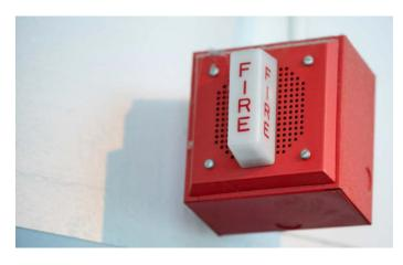
Fire alarm notification appliances, such as audible alarms and visual emergency signals (e.g. horns, buzzers, flashing lights), can also provide alternative pathways for power surges to enter the FACP. These devices are all connected to the FACP via Notification Alarm Circuits (NACs) and monitored via Initiating Device Circuits (IDC) within the FACP. Protecting these devices and FACP circuits will protect the fire alarm and life safety system from possible power surge points of entry.
