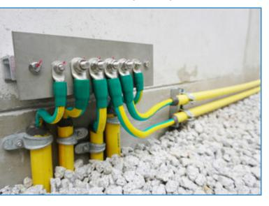
diverted to earth through the facility's electrical grounding system, so a low-resistance grounding system is a key component for the facility's surge protection strategy.
