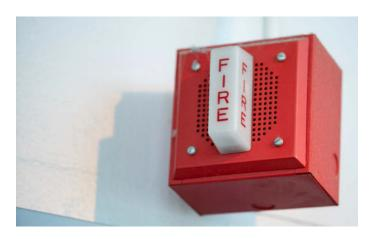
Fire alarm notification appliances, such as audible alarms and visual emergency signals (e.g. horns, buzzers, flashing lights), can also provide alternative pathways for power surges to enter the FACP. These devices are all connected to the FACP via Notification Alarm Circuits (NACs) and monitored via Initiating Device Circuits (IDC) within the FACP. Protecting these devices and FACP circuits will protect the fire alarm and life safety system from possible power surge points of entry.
