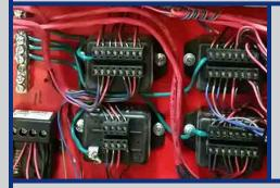
When installing multiple SPD's and terminating to a common electrical ground, a dedicated ground wire running from each individual SPD to a common grounding bus bar is strongly recommended. "Daisy-chaining" multiple SPD ground wires together via the SPD grounding terminals, or by using twist-on wire connectors, is not recommended as this increases the resistance and extends the length of the ground path.
