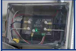
Whenever possible, Surge Protective Devices should be installed in a dedicated enclosure outside of the equipment being protected. This will prevent physical damage to the electronic circuit board, power supply and/or wiring inside of the equipment panel due to a potential catastrophic failure of the SPD.
