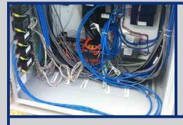
The conductor length between the SPD and the equipment being protected should be a minimum of 3 feet in length to allow enough time for the SPD to react. The conductors can be greater than 3 feet as long as they are isolated and are not subjected or directly exposed to internally- or externally-generated transient voltage spikes and/or surges.
